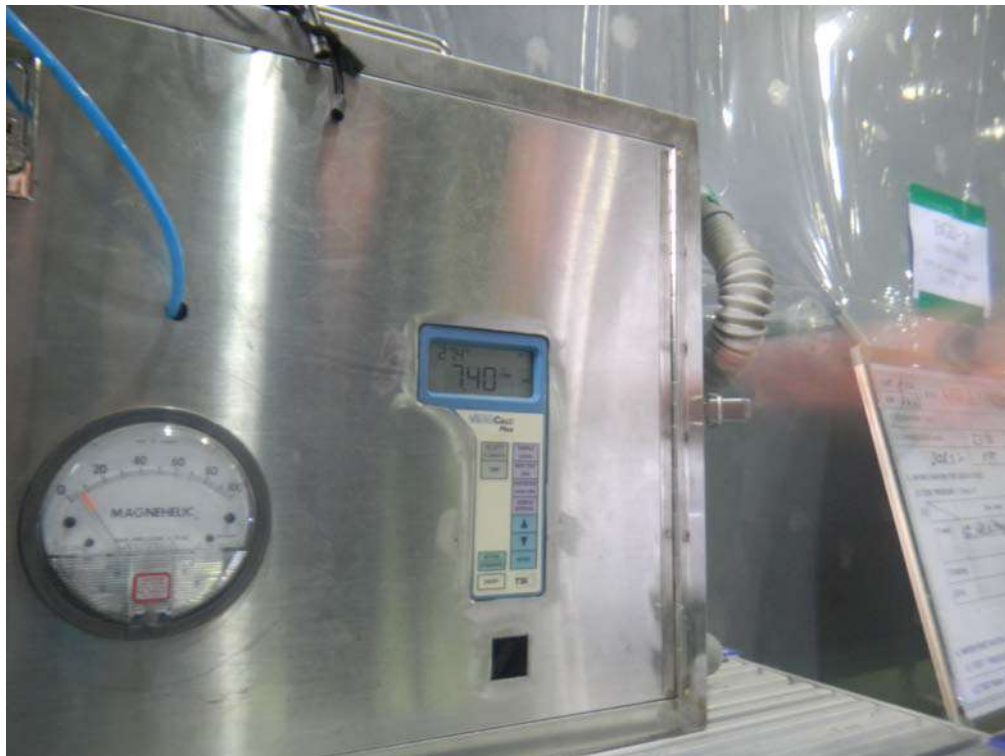
<photo> air leakage test<BGD - 2>
