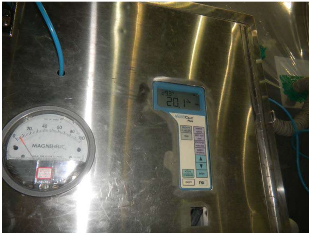
<photo> air leakage test <BGD - 8>
